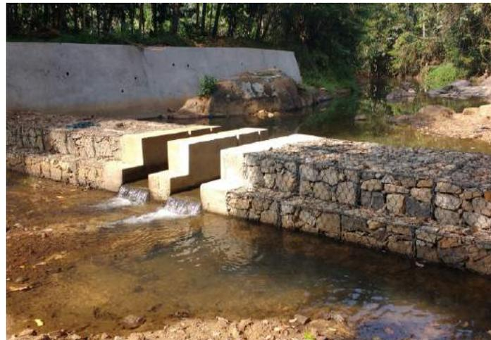
*Figure 4. Gabion Check Dam*
