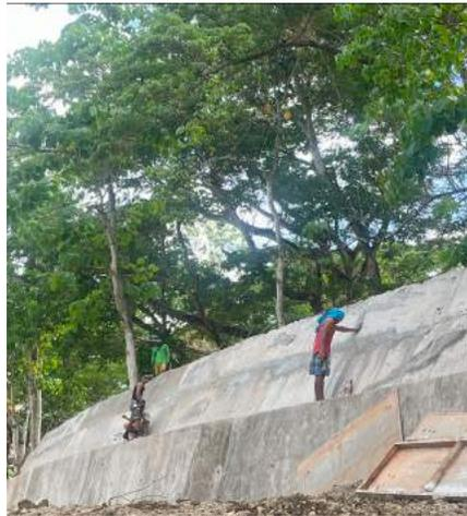
*Figure 1. Height of the riprap wall, human person for scale*
